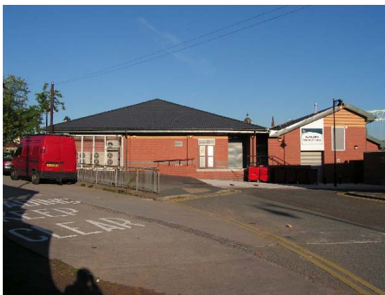
View of Alcock Street 'service yard' from bus station.
