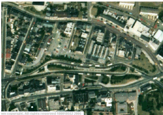
Aerial view of Central Area in 1983 showing the elaborate busway interchange severing linkages between Church Street (top) and High Street (bottom).
