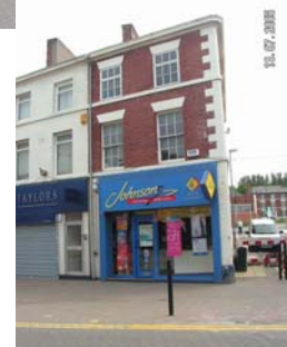
Church Street South side unit with non- standard Frontage treatment
