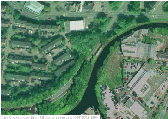
Aerial view of section of busway running parallel to north bank of Bridgewater Canal between Bridge Street and Leiria Way and former Petrol Filling Station that may be suitable for future housing development.
