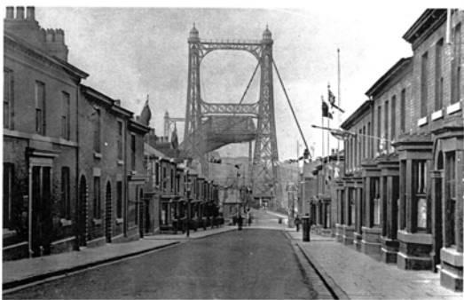
View of the approach to the Transporter Bridge, which provided the sole vehicular link between Runcorn and Widnes until 1961.
